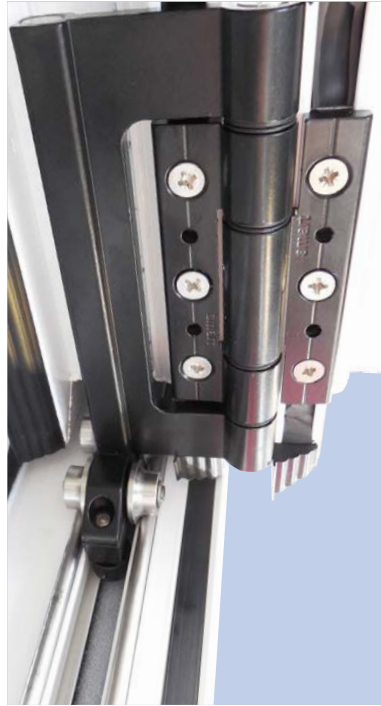
View of retained roller hinge
