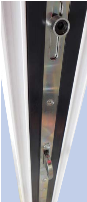
View of lower hook bolt and cam
