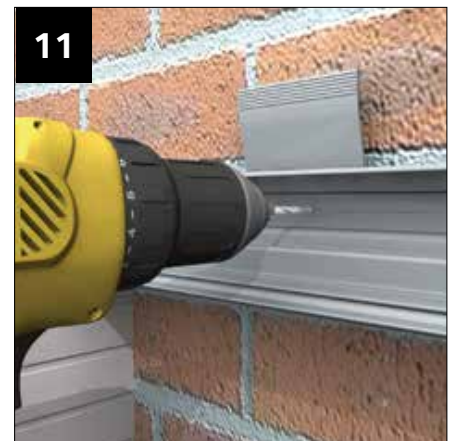
11 Drill through the wallplate main body and directly through each carriage to suit the masonry anchors being used (not supplied). Mark the position of each masonry anchor on the house wall and drill the house wall to suit.
