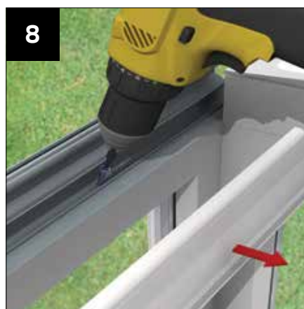
8 Drill a 5mm pilot hole in the head of the frame, fasten down using 4.8 x 32mm screws (not supplied) at 450mm centres. Refit internal claddings. If fastening up through the frames into the eaves beam use 4.8 x 55mm screws.
