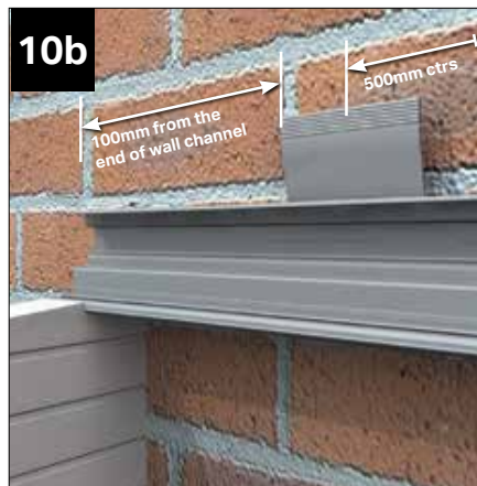
10b Offer the wallplate up to the wall and position it so that the top surface of the bolt slot is level with the top of the firrings.
