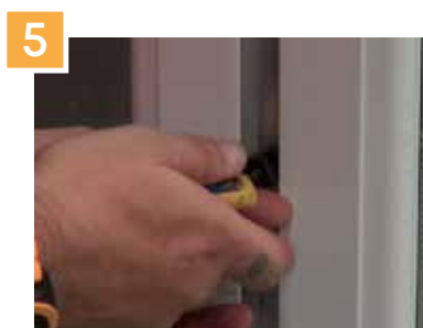
5 Rotating the 1/4 turn button with an Allen key secures the panels and ensures they are the correct distance apart.
